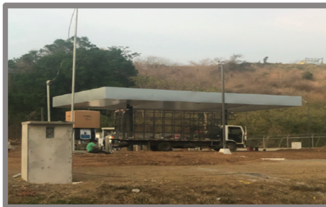
Picture E-15-Gas Station Construction Site in Playa Veano
