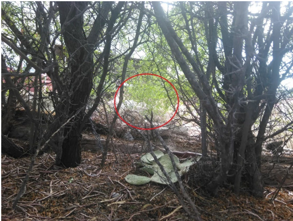
Image of the hole (circled in red) cut in the back fence at the Sierra Mojada Project Camp Site, June 2020.
