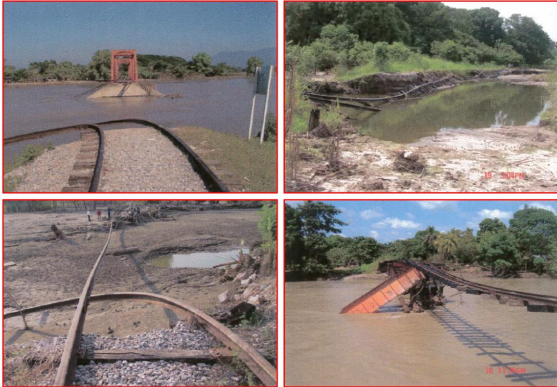
Image 8: Pictures of the damage caused by Hurricane Stan in the Chiapas Line (C-69-SPA)
